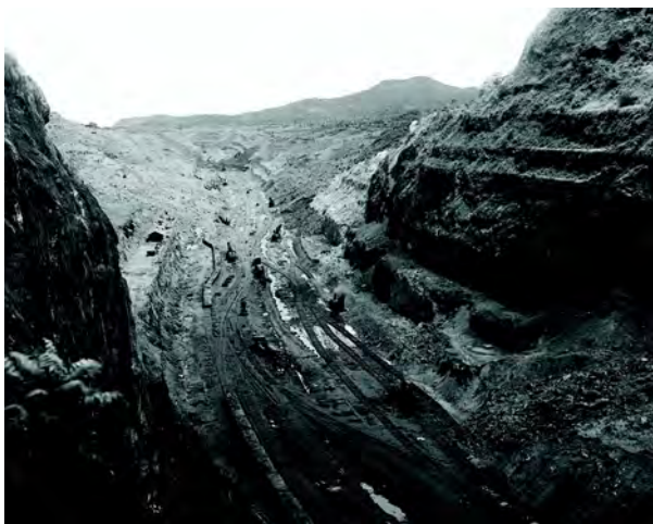
Culebra Cut during excavation
