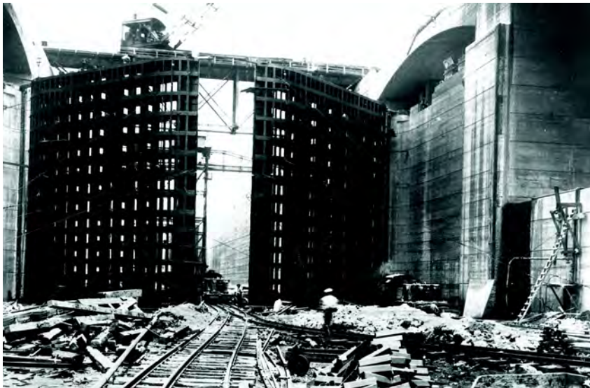
Miraflores lock under construction
