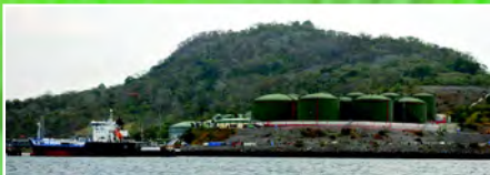
Taboguilla Island bunker terminal
