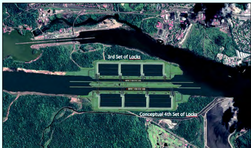
Aerial view showing placement of locks
